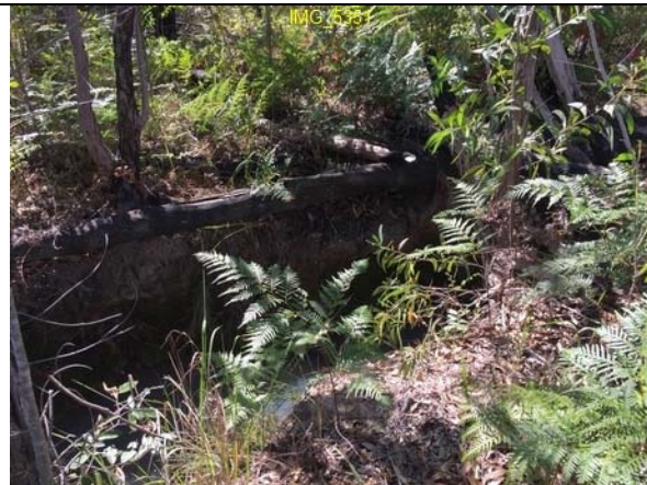
CH900-1000 narrow incised low flow channel (1m wide to 0.75m deep) alternating with grassed broad sheet flow area, small pockets of scour pool, generally good vegetation cover outside low flow channel.
