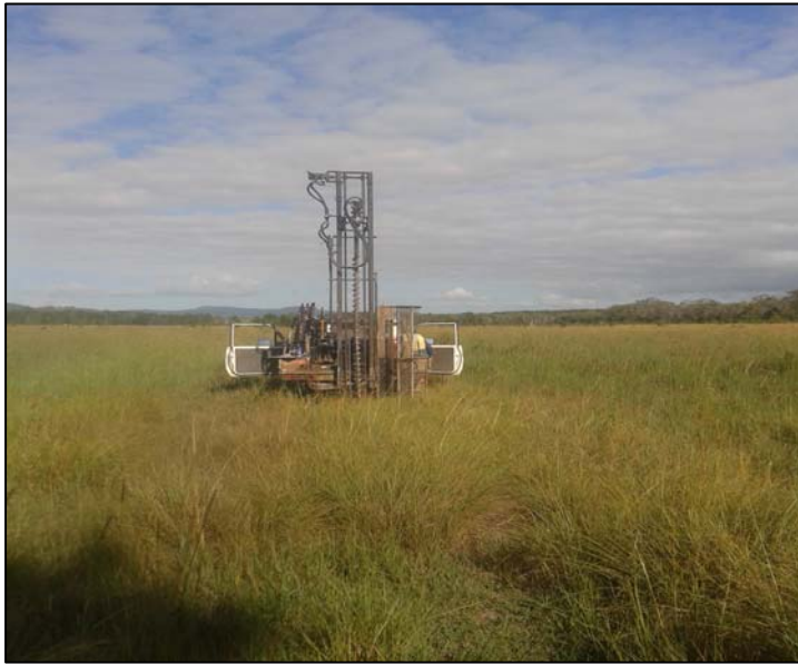
Figure 1: Typical site conditions for Precincts 7 – 15
