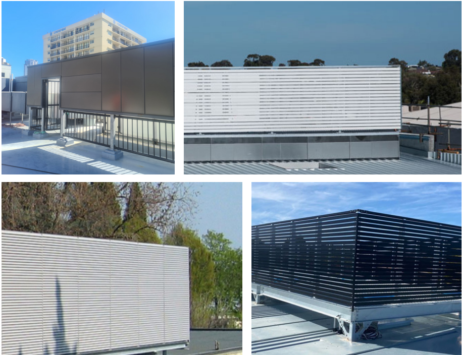
A/C PLANT FENCING TREATMENT | MONDRIAN OF DIFFERENT SCALE LOUVRES TO CREATE VISUAL INTEREST TO THE A/C ENCLOSURE TO BE FURTHER DETAILED IN DESIGN DEVELOPMENT PHASE.
