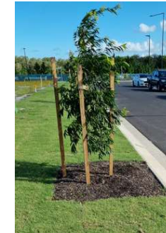
ADDITIONAL TREE STAKE ARRANGEMENT TO AID TREE PROTECTION
