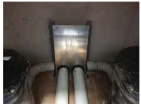
Figure 3 - Typical Outlet Weir Wall
