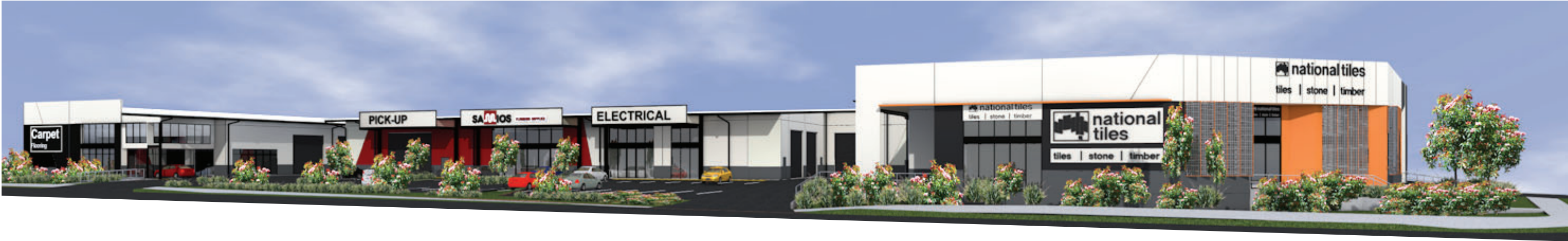
01 South East View - Carnegie Street
