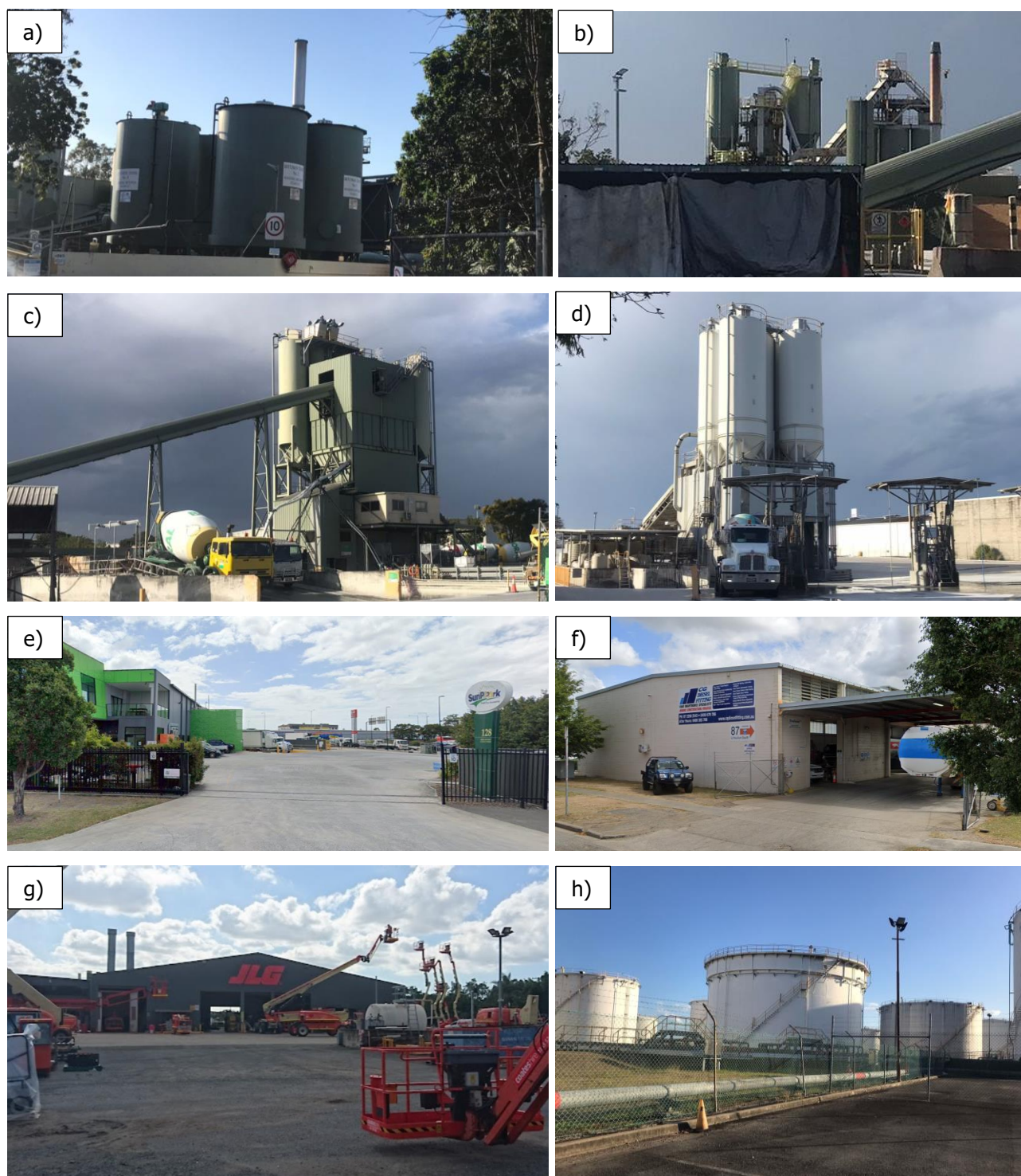
Figure 3.4 Front view of industries identified surrounding the proposed development: BCC Asphalt & Aggregates; b) Boral Asphalt; c) Boral Concrete; d) Holcim Concrete; e) SunPork Fresh Foods; f) CQ Diesel Fitting; g) JLG Industries; h) BP Whinstanes Terminals
