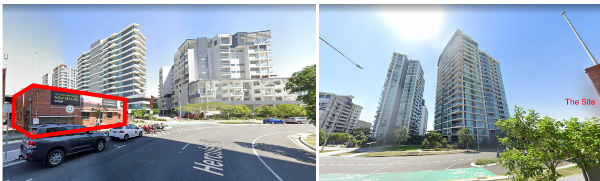
Figure 7: Existing context to the south and west of the site
