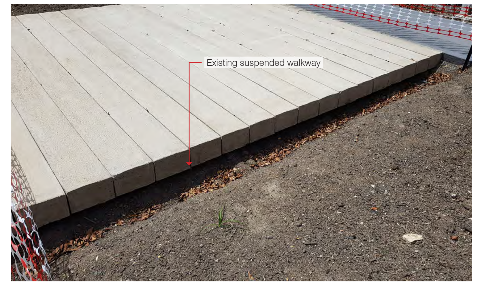
Existing suspended walkway
