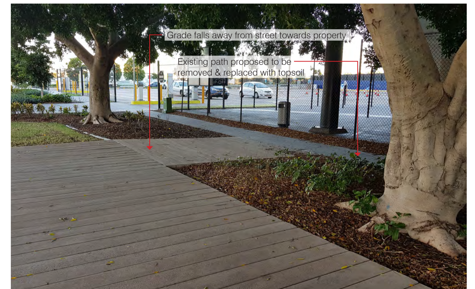
Existing suspended walkway
