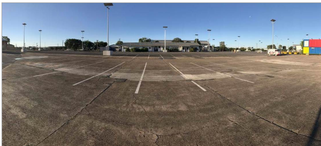
Photograph 2: Panoramic view of part of the site looking north from near Blockyard Spaces towards Blockyard Workshops with Eat Street Northshore visible in the right hand side of the photograph
