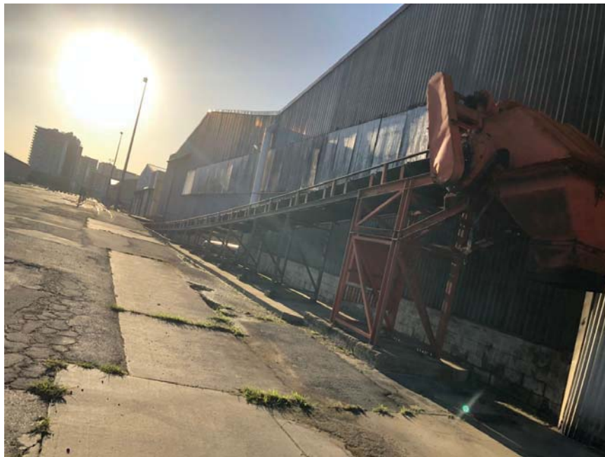
Photograph 4: Photograph of the northern warehouse and conveyor belt taken along the central area of the site towards the west.
