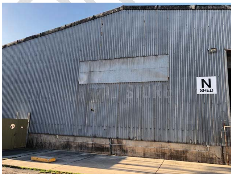
Photograph 22: View of N shed with faded 'bulk mineral store' sign
