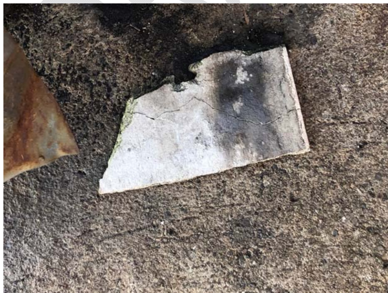
Photograph 20: View of possible asbestos roof tile, identified at surface near BH10
