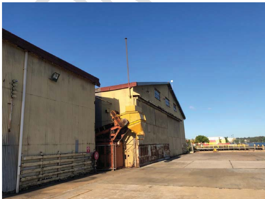
Photograph 24: View of historical mineral sand loading point
