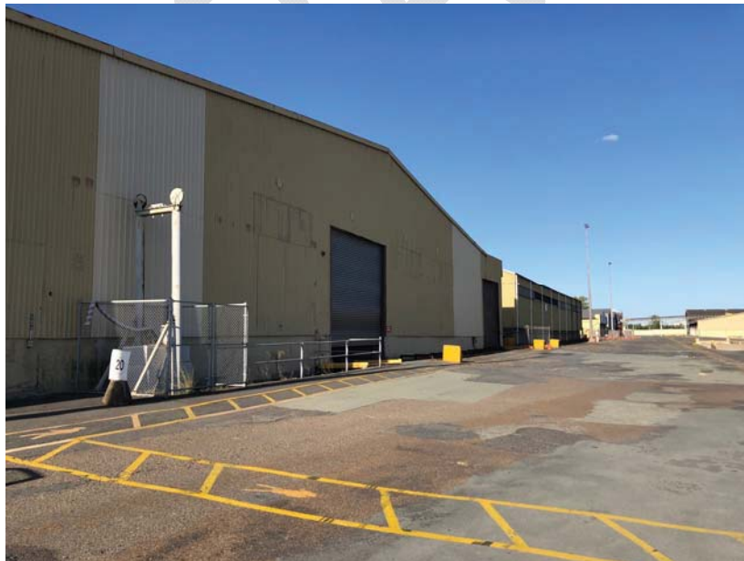
Photograph 3: Photograph of the northern warehouse taken along the central area of the site towards the east.
