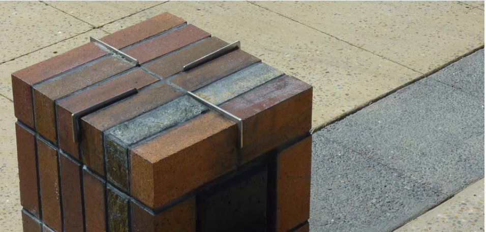
BOLLARD TYPE 1 HOSTILE VEHICLE MITIGATION BOLLARD
