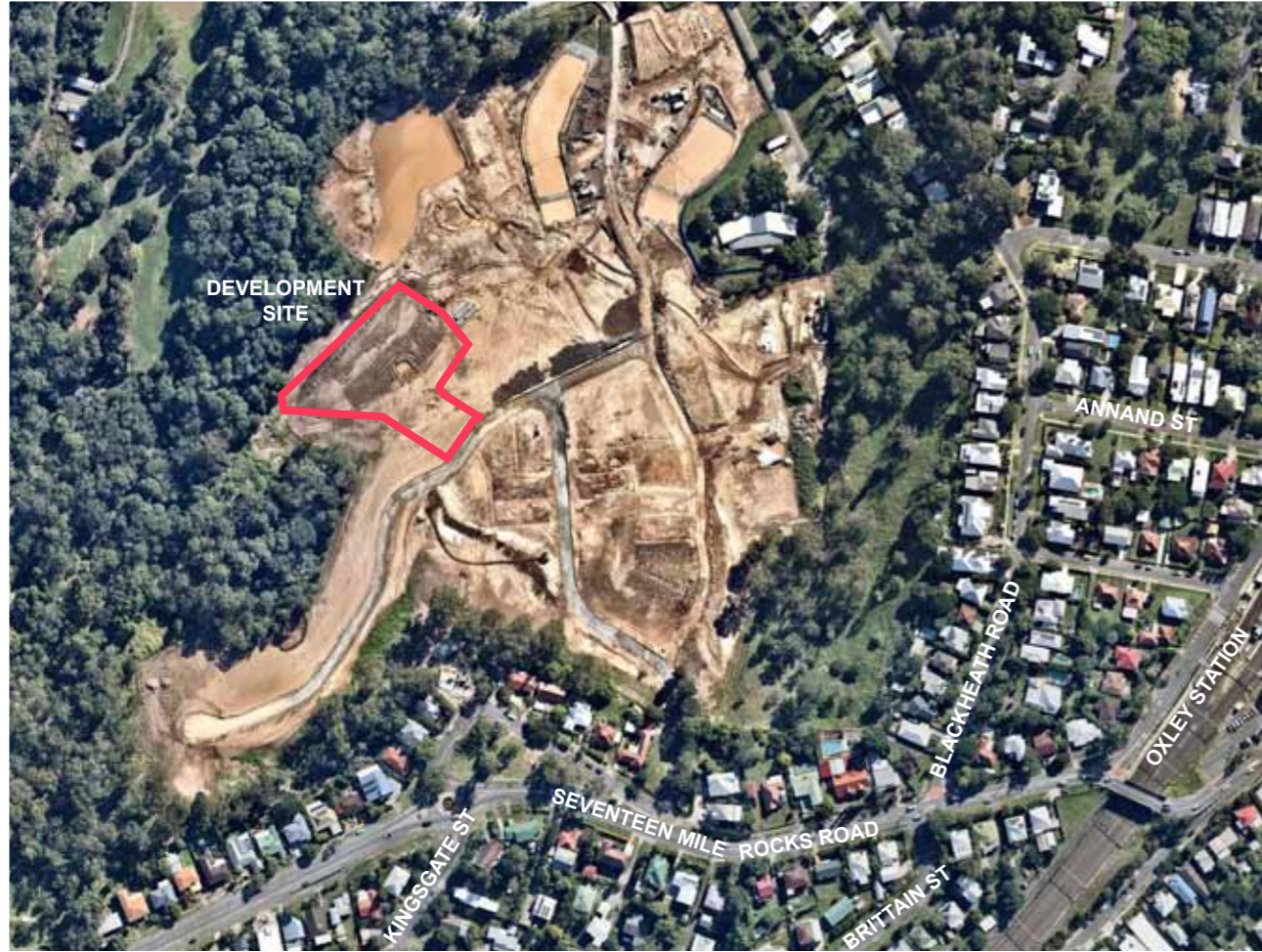
Aerial photograph of existing site extent
