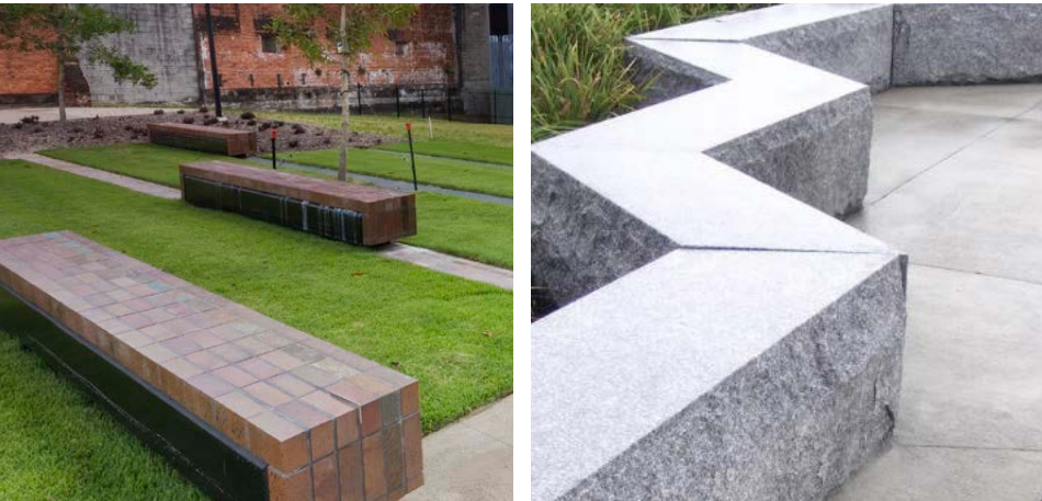
SEAT TYPE 1 ST1 - PRECAST CONCRETE WITH STONE / BRICK FACING
