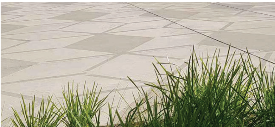
Concrete Sandblasting
