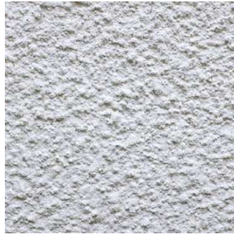
TEXTURED CONCRETE RENDER
