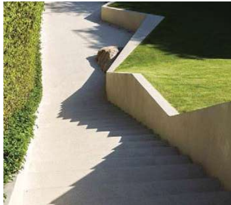
Concrete planter walls
