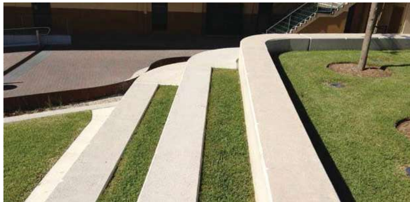
Cast insitu concrete terraces
