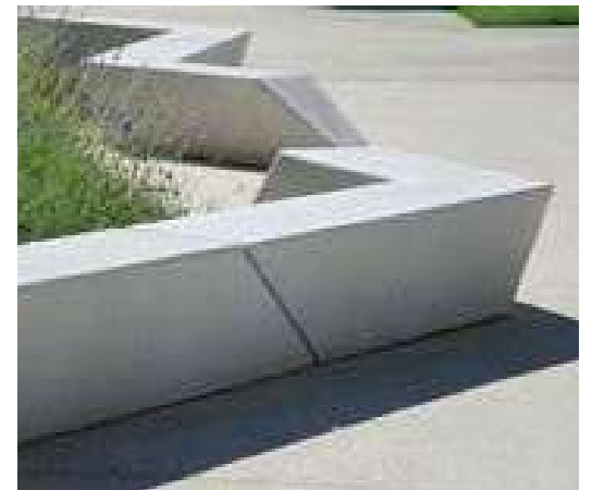
Cast insitu concrete seats
