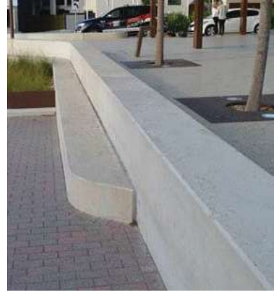
Formed Concrete Seating Element RNA Showgrounds
