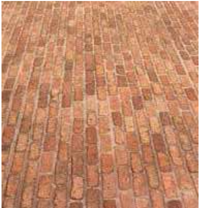
A strong banding pattern is reinforced by introducing red brick into large expanses of paving, specifically near focal points
