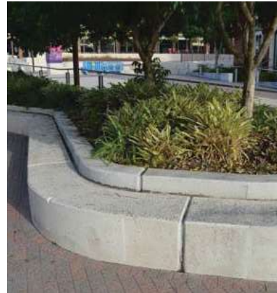
Formed Concrete Seating Element Example: RNA Showgrounds
