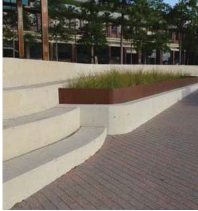
Formed Concrete and Weathered Steel Planters RNA Showgrounds
