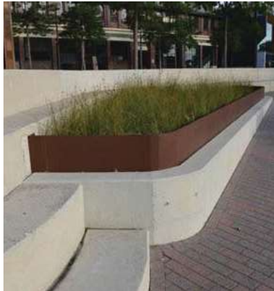
Formed Concrete and Weathered Steel Planters Example: RNA Showgrounds
