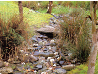
Planted dry creek bed and grass swales will be used to convey overland flow through the lower section of the pocket park
