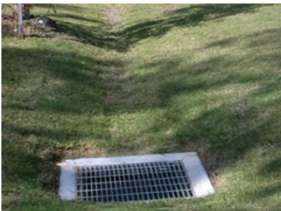
Planted dry creek bed and grass swales will be used to convey overland flow through the lower section of the pocket park
