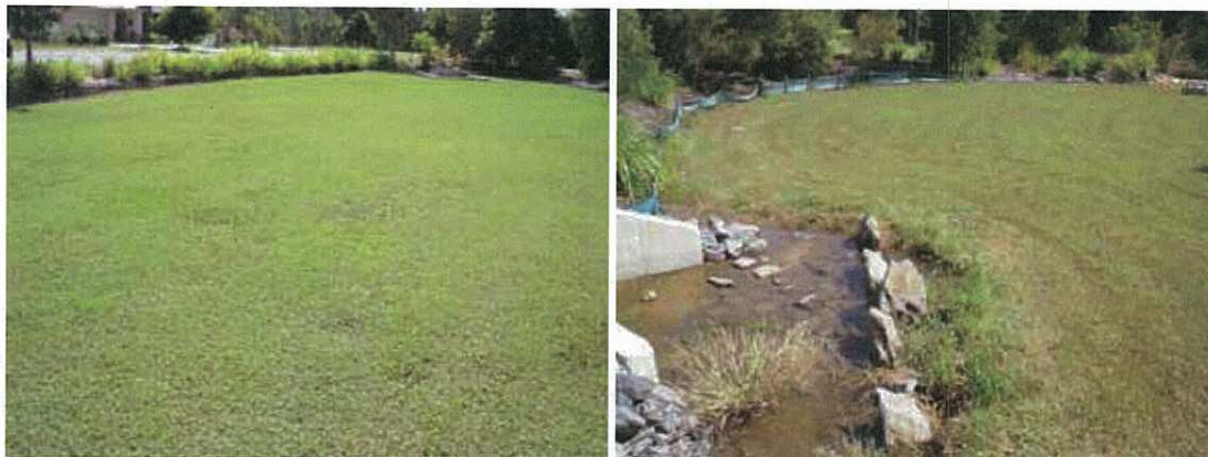
Figure 3-5 Example of a Bioretention Basin with Temporary Protection (During Lot-Scale Works)
