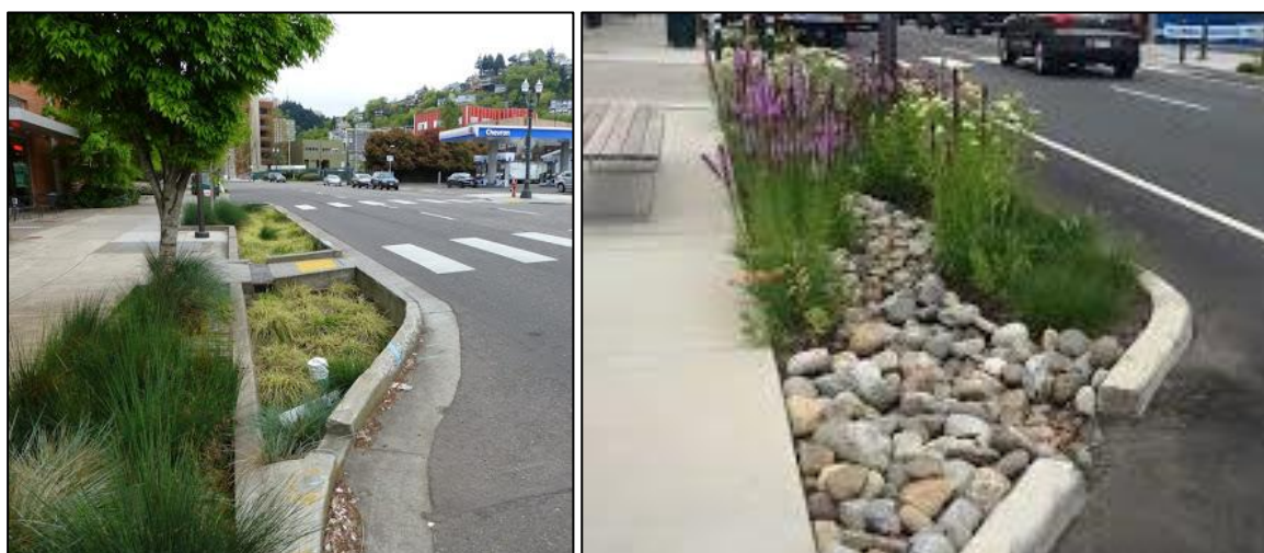
Figure 2.4 Indicative Bioretention Pod Design
