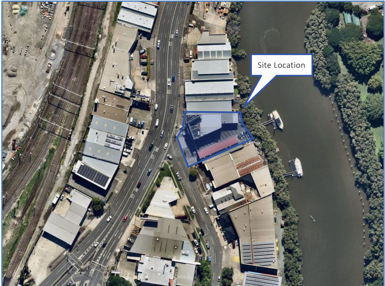
Figure 1-2: Site location (Source: Nearmap)
