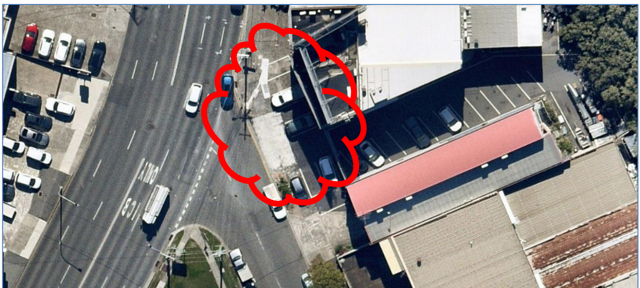
Figure 1-4: Existing Parking Provisions (Source: Nearmap)
