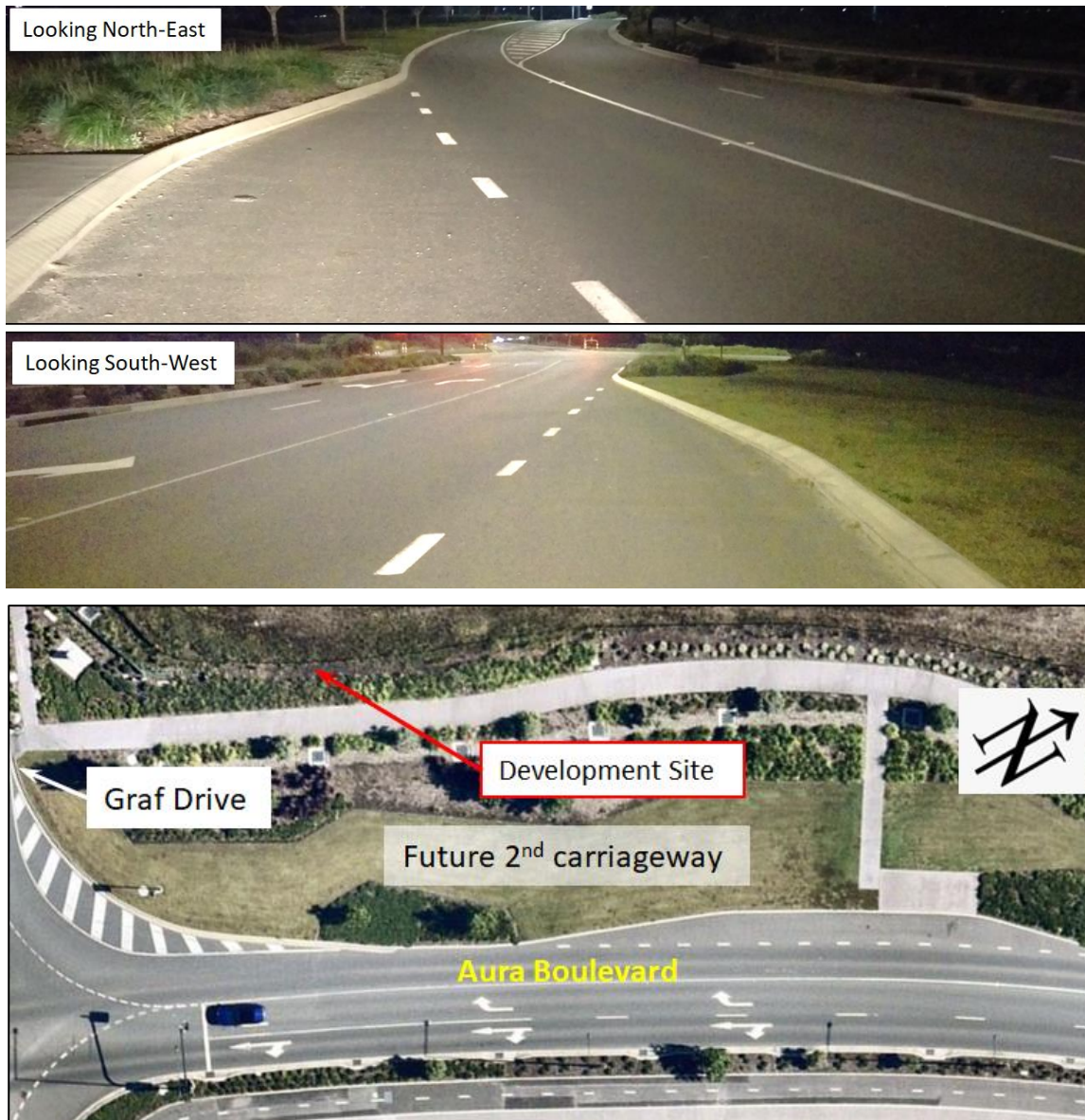
Figure 2-4 Aura Boulevard (Source : Nearmap)
