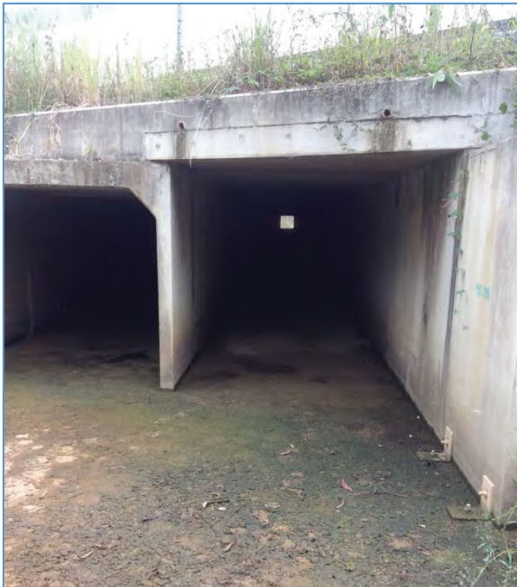
Figure 6 Photos of culverts under the Mount Lindesay Highway, showing a) rock scour protection upstream of culvert apron, b) rocks and ponded area with Typha downstream of culvert, c) the culverts are long and dark, and d) possible low-flow channel incorporated into design of culverts.
