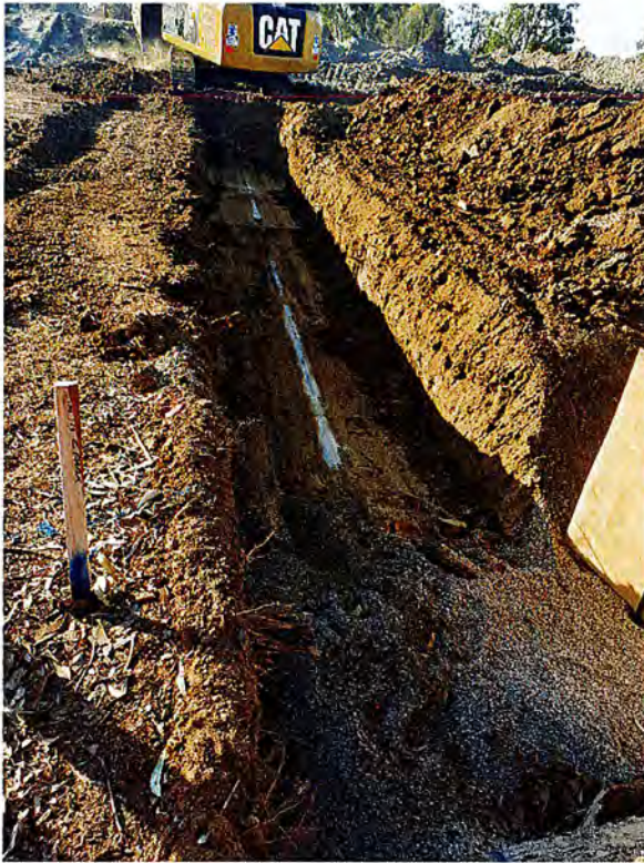
Plate 1: Redundant Stormwater Pipe within Stage 1
