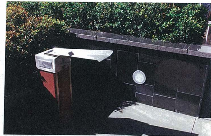
Paving and ground surface treatments wrapping up podium walls providing a continuation and integration of materials
