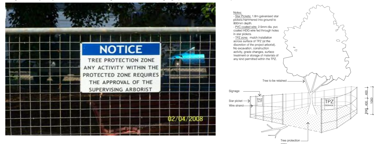
Image 3 – Temporary Metal Exclusions Fencing and Exclusion Zone Signage (Source Arbor Australis)
