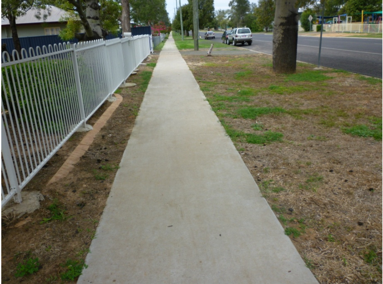
Figure 2.4: Concrete Footpath on the Northern Side of McDowall Street
