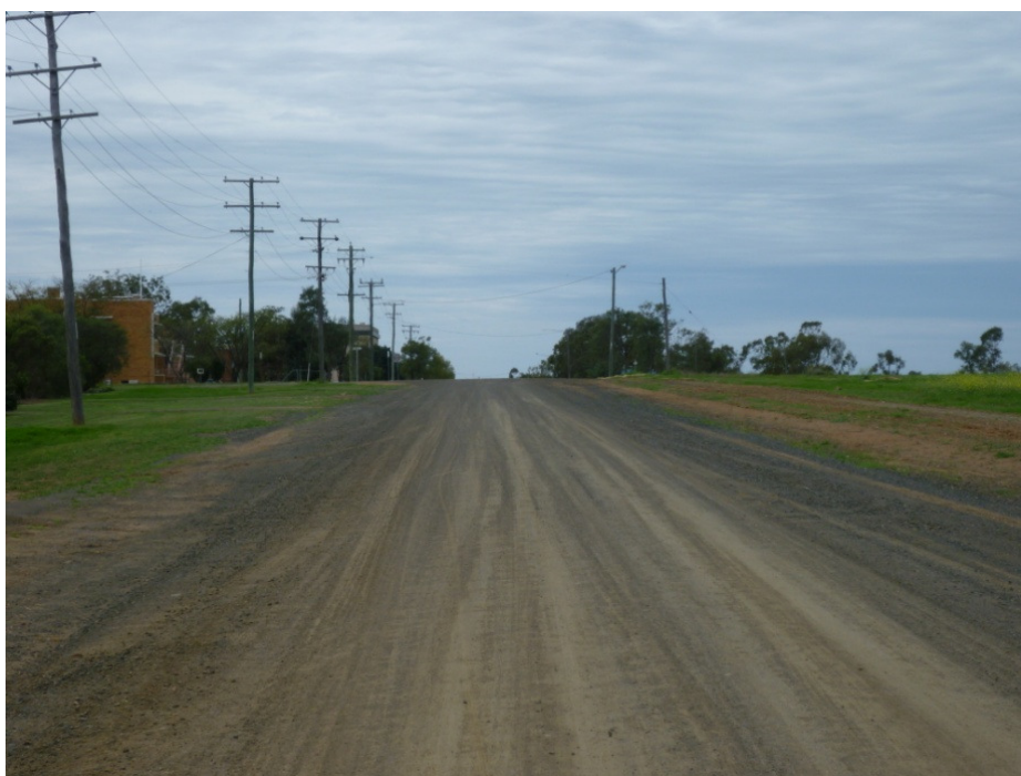
Figure 2.1: Unsealed Stretch of McDowall Street
