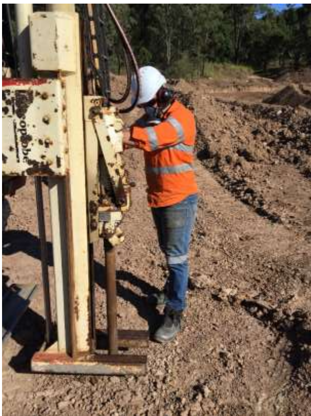
Figure A1 Field works in progress
