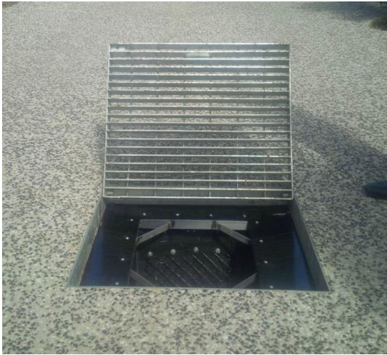
Figure 4-1 Example SPEL Stormsack in Field Inlet Arrangement.
