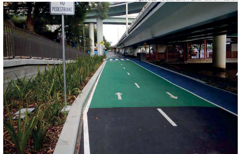
Figure 5.53: Existing Transition Zone A Conditions
