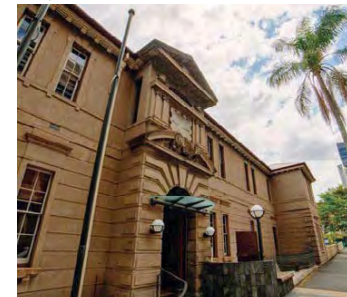
Former DPI Building entrance
