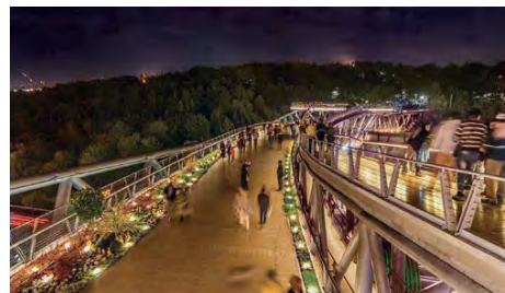
Suitable bridge widths are important to provide for comfortable pedestrian flows
