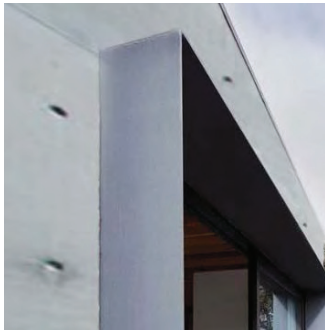
GLAZED OPENINGS EXPRESSED BLACK STEEL LINTELS
