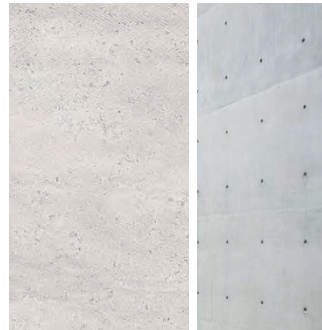
EXTERNAL WALLS EXPOSED & TEXTURED CONCRETE
