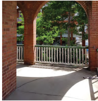
E BLOCK & TOWERS CONCRETE VERANDAH - REPAIRED WHERE NECESSARY
