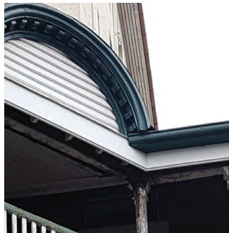
GT 1 GUTTERS TO E BLOCK & TOWERS NEW PAINT TO MATCH EXISTING
