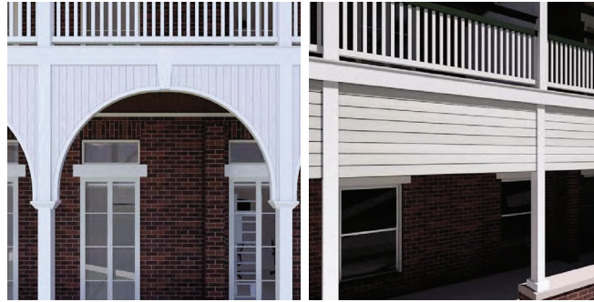
PT 3 WHITE PAINT TO ALL TIMBER WORK NEW PAINT TO MATCH EXISTING
