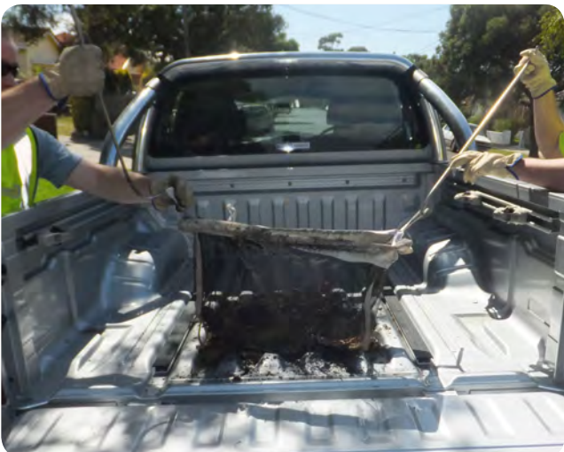
Photo 16 Grab the bottom lifting loops
