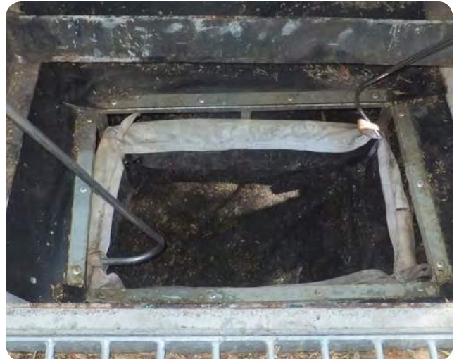
Photo 21 Correctly installed filter bag
