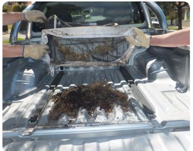
Photo 17 Lifting the bottom bag loops empty the filter bag
