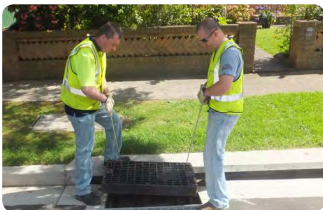
Photo 9 Lift grate above the support frame
