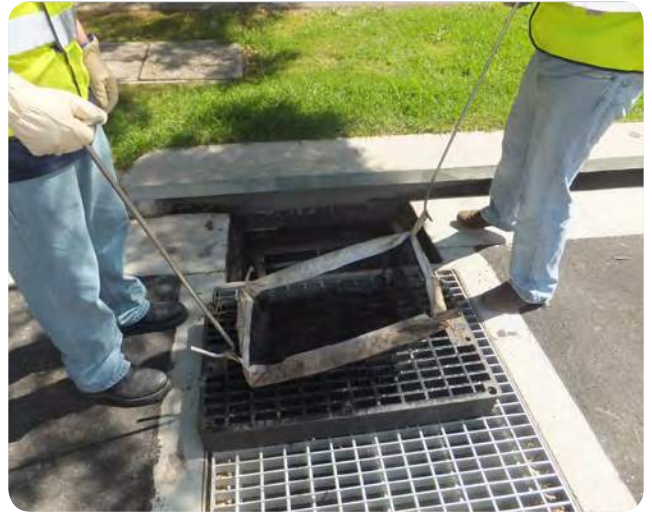
Photo 19 Reinstall filter bag
