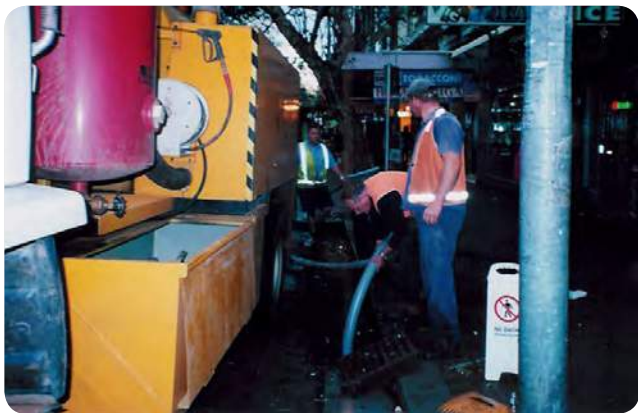
Photo 11 Cleaning an EnviroPod using the inductor method
