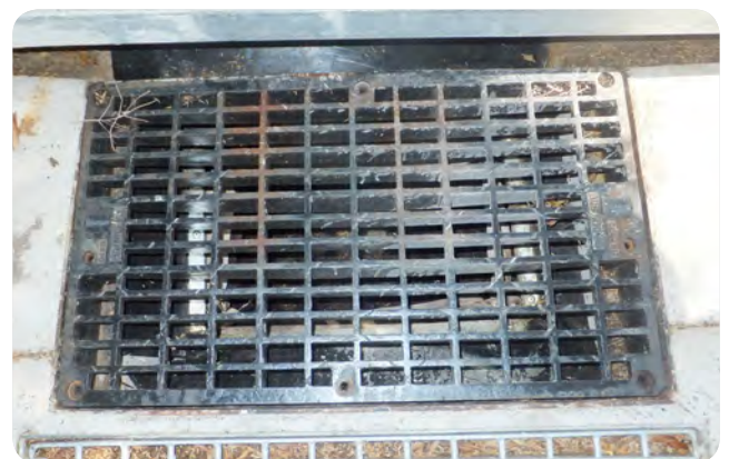
Photo 10 Reinstated non hinged grate
