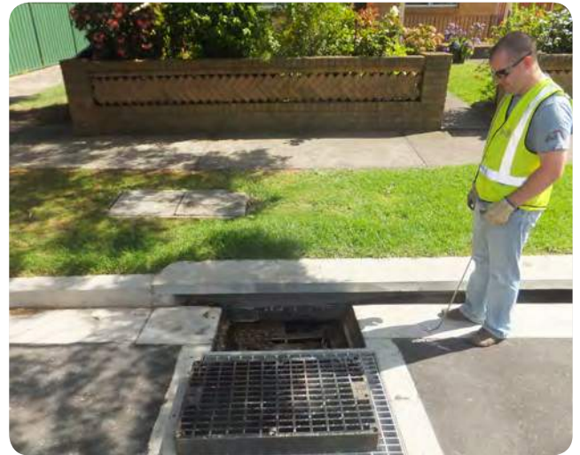
Photo 4 Fully open grate
