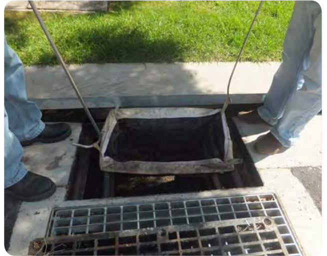
Photo 13 Lift the bag from the cage and support frame
