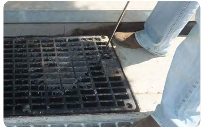
Photo 6 Insert hook near edge of grate
