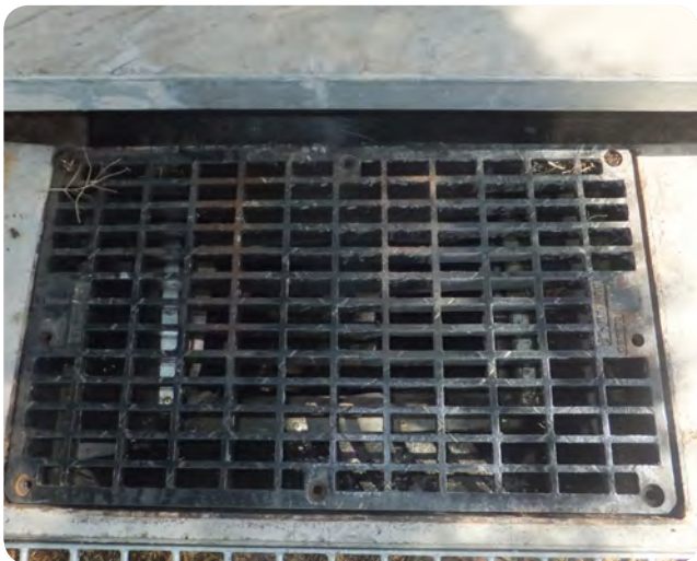
Photo 22 Installed filter bag and sealed pit
