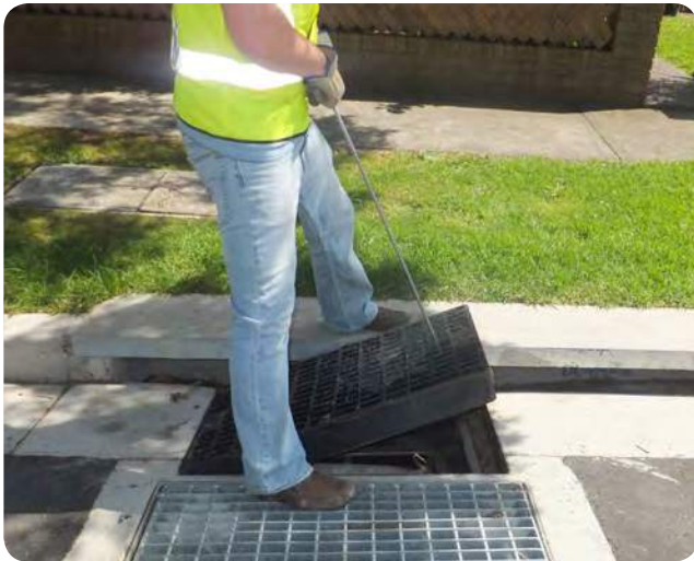
Photo 3 Lifting the grate
