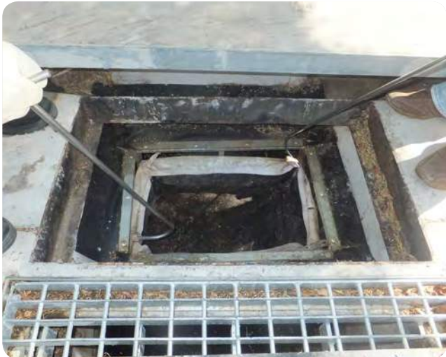
Photo 20 Ensure that the unit is positioned correctly, with the lifting loops on the inside
