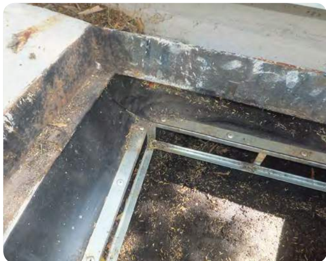
Photo 23 Check seals are pushed against the pit walls
