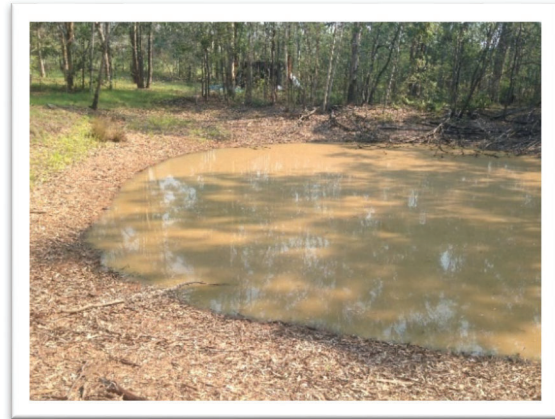
Plate 4. View of existing earthen base dam with dense leaf littered banks.
