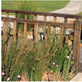
BRIDGE CROSSING WITH HANDRAIL
