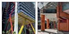
High quality finish to the surface of columns, with column form, material and colour forming part of the overall building facade
