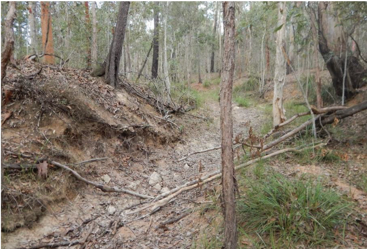
Figure 4.1: Existing Eroded Creek Line within the Site
