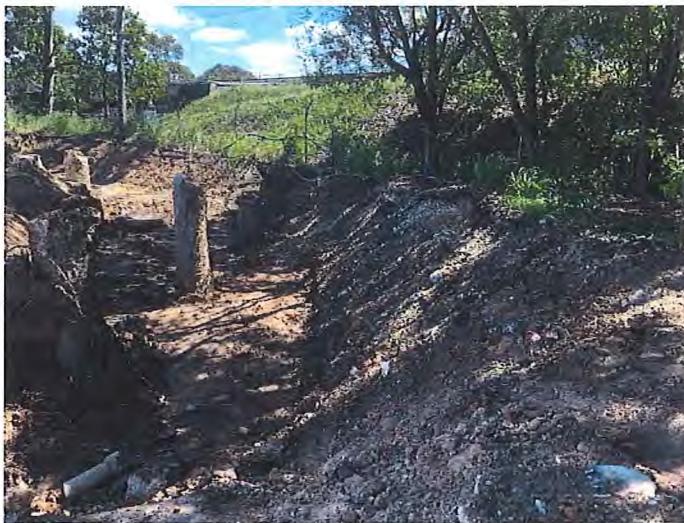
Photograph 3: A view of the northern vegetated portion of the site facing towards the west, with the bund material that contains C&D Waste and ACM pictured in the right of the photograph. (Image Date: 3 July 2019)
