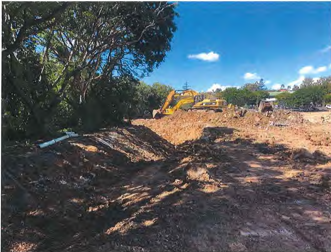
Photograph 4: A view facing towards the east during waste removal works, with the bund and northern vegetated portion of the site visible in the left of the photograph. (Image Date: 4 April 2019)
