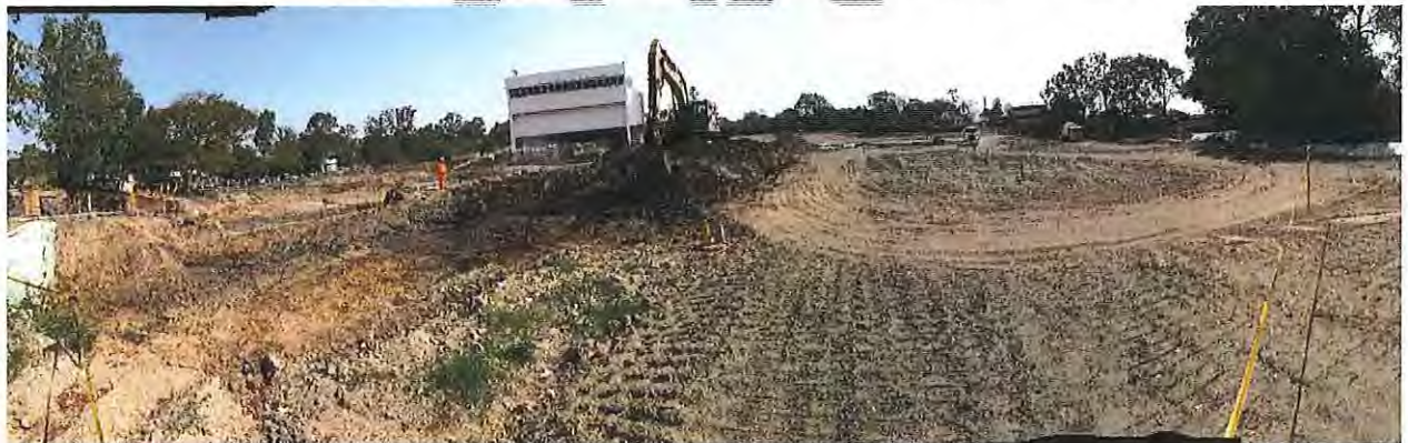
Photograph 5: A panoramic view of the northern portion of the site after the conclusion of filling works, the northern vegetated portion of the site is visible with geofabric placed on the bund material pictured in the top right of the photograph. (Image Date: 9 October 2019)
