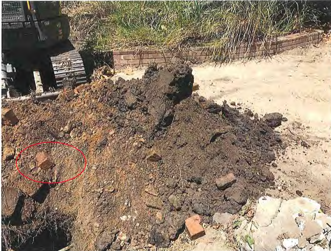
Photograph 1: An example of C&D Waste (circled in red) found in Test Pit (TP-N5) within the northern vegetated portion of the site. (Image Date: 3 December 2019)
