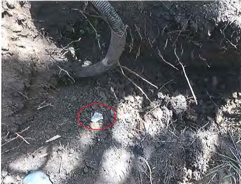
Photograph 2: An example of ACM (circled in red) found in Test Pit (TP-N8) excavated in the northern vegetated portion of the site. (Image Date: 3 December 2019)
