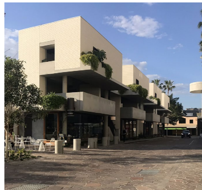
PAVEMENT TREATMENT PROMOTES SLOW AND SHARED PEDESTRIAN ZONE.
