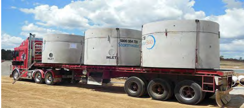
Figure 4: Pre-cast concrete manholes
