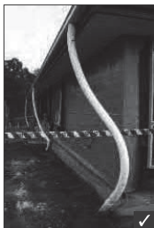
Temporary roof water connection
