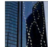
Encourage night time economy by employing quality lighting outcomes and creative expression of lighting that together contribute to building design and identity
