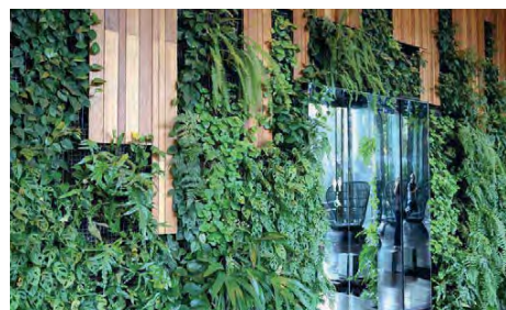
Green walls help soften architectural forms
