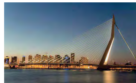
The bridge provides a direct pedestrian connection between the City and South Bank
