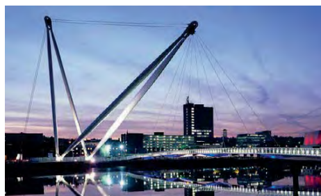
The design response is proposed as a dramatic, slender, arch-like structure that will be a vertical beacon along the river's edge
