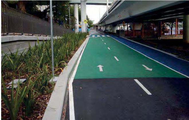
Figure 5.37: North Quay Existing Bikeway Conditions
