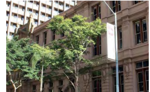
The Printery Building and existing streetscape
