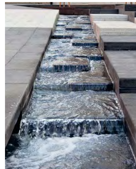
Utilise cascading water features at the Brisbane Steps to cool, and mask noise.
