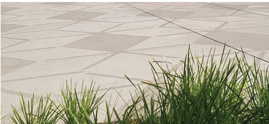
Concrete Sandblasting
