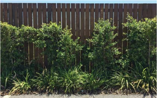
TIMBER PALING FENCE TO CARPARK PERIMETER (1800mm HIGH)
