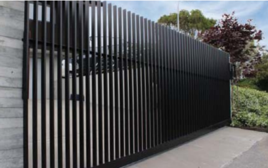
ALUMINIUM BATTEN FENCE TO OUTDOOR PLAY AREA (1800mm HIGH)
