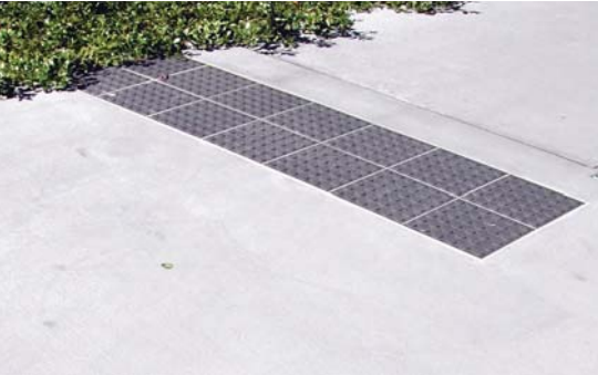
PLAIN BROOM-FINISH CONCRETE PATHS WITH BCC STANDARD TACTILE SURFACE GROUND INDICATORS (TGSi)
