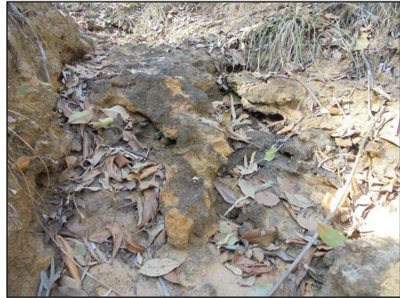
Image 6. Tunnel erosion within drain bed
