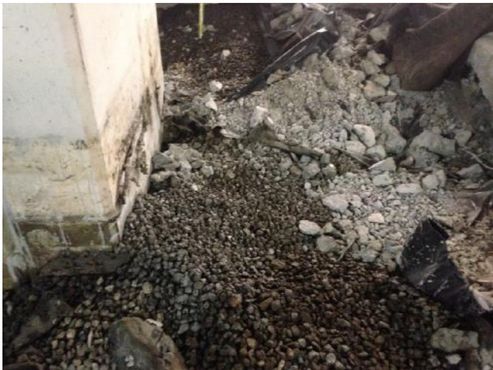
Photo 4 – Drainage Layer Material under slab
