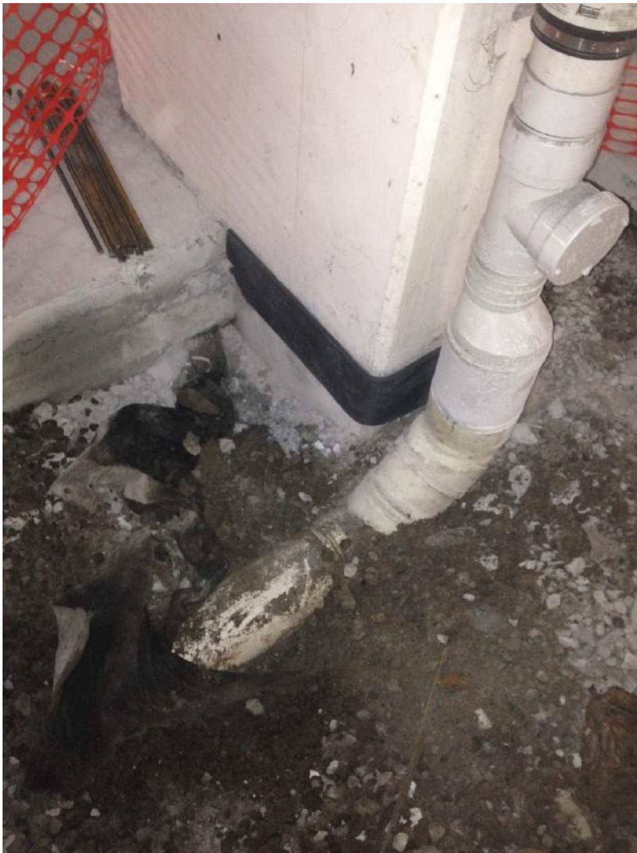
Photo 5 - Existing sewer pipe not broken
