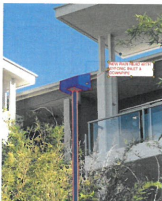
TYPE 1: RAINHEAD – BALCONY ACCESS NOT TO SCALE
