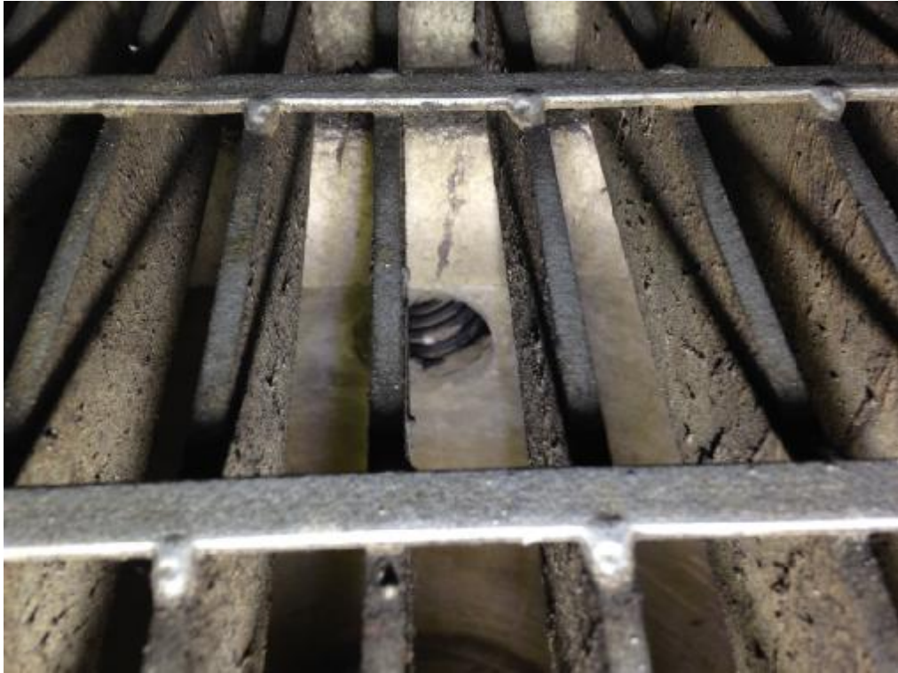
Photo 3 – Grated Inlet Pit on basement drainage system – 50mm ag drain from under slab drainage layer can be seen
