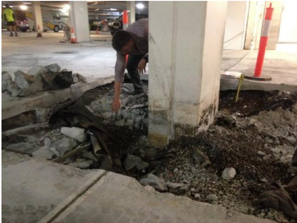
Photo 3 – General photo of excavation with void, drainage layer and geofabric visible
