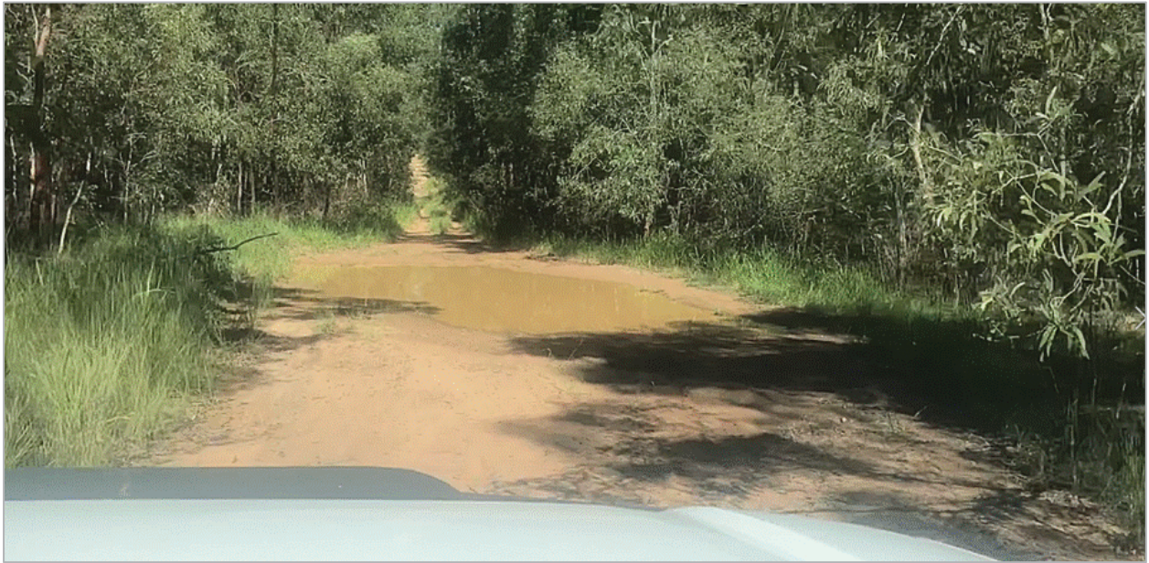
Figure 4.2 Teviot Road (west) Typical Existing Condition
