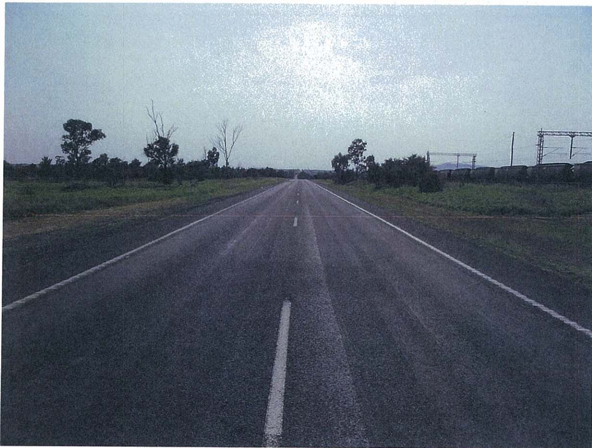
Photo: 1 Capricorn Highway looking east
