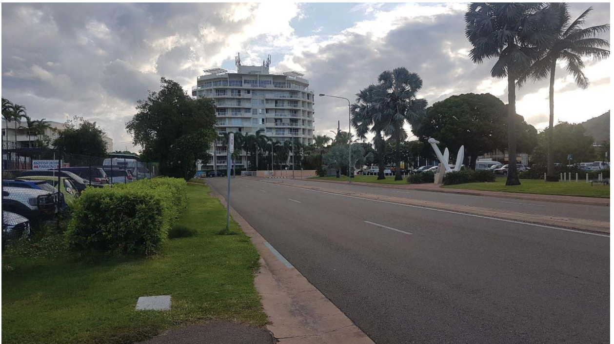
Figure 5-9: Sir Leslie Thiess Drive looking South from the proposed left-in left-out access
